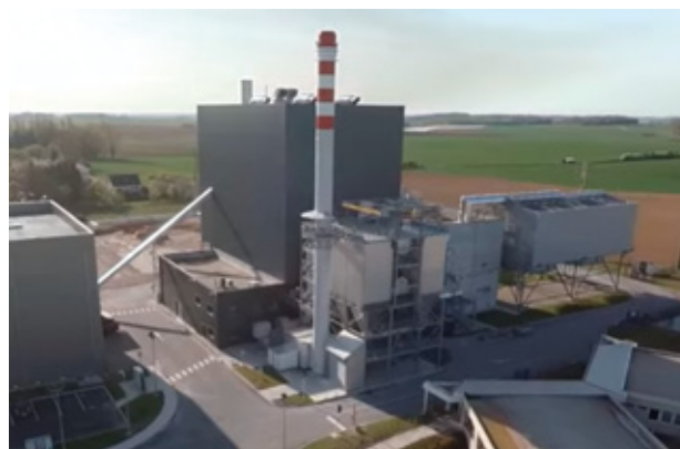
Biomass boiler recovering wood waste from a local forestry operation and supplying steam to the Bonduelle plant in Estrées-Mons (France).
