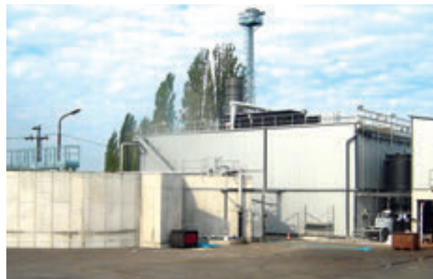
WASTE WATER TREATMENT FACILITY Békéscsaba plant in Hungary.
